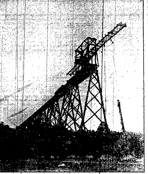
BUILDING THE RICHLAND CREEK VIADUCT. The largest transportation structure in the world...
